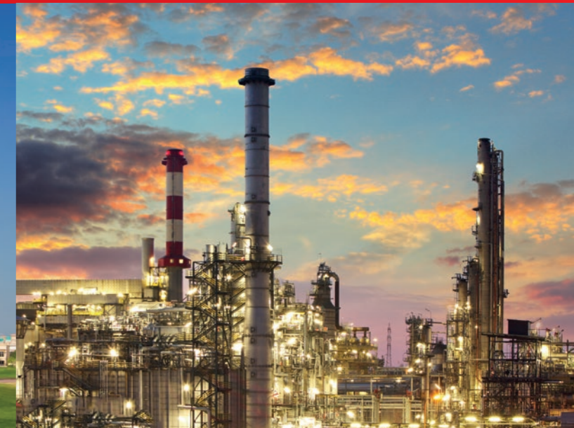
Petronas Refinery, Kuala Lumpur, Malaysia
