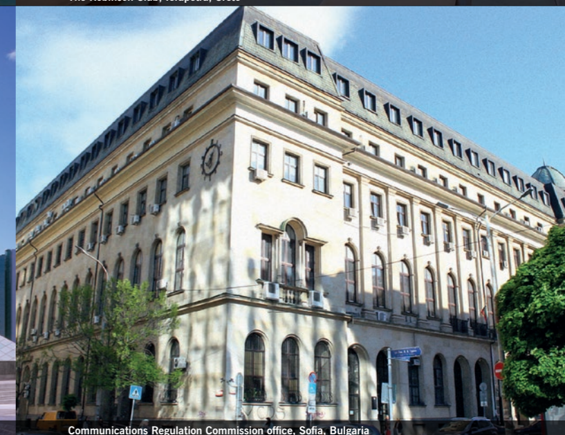
Communications Regulation Commission office, Sofia, Bulgaria
