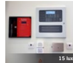
Fire alarm control and indicating equipment
