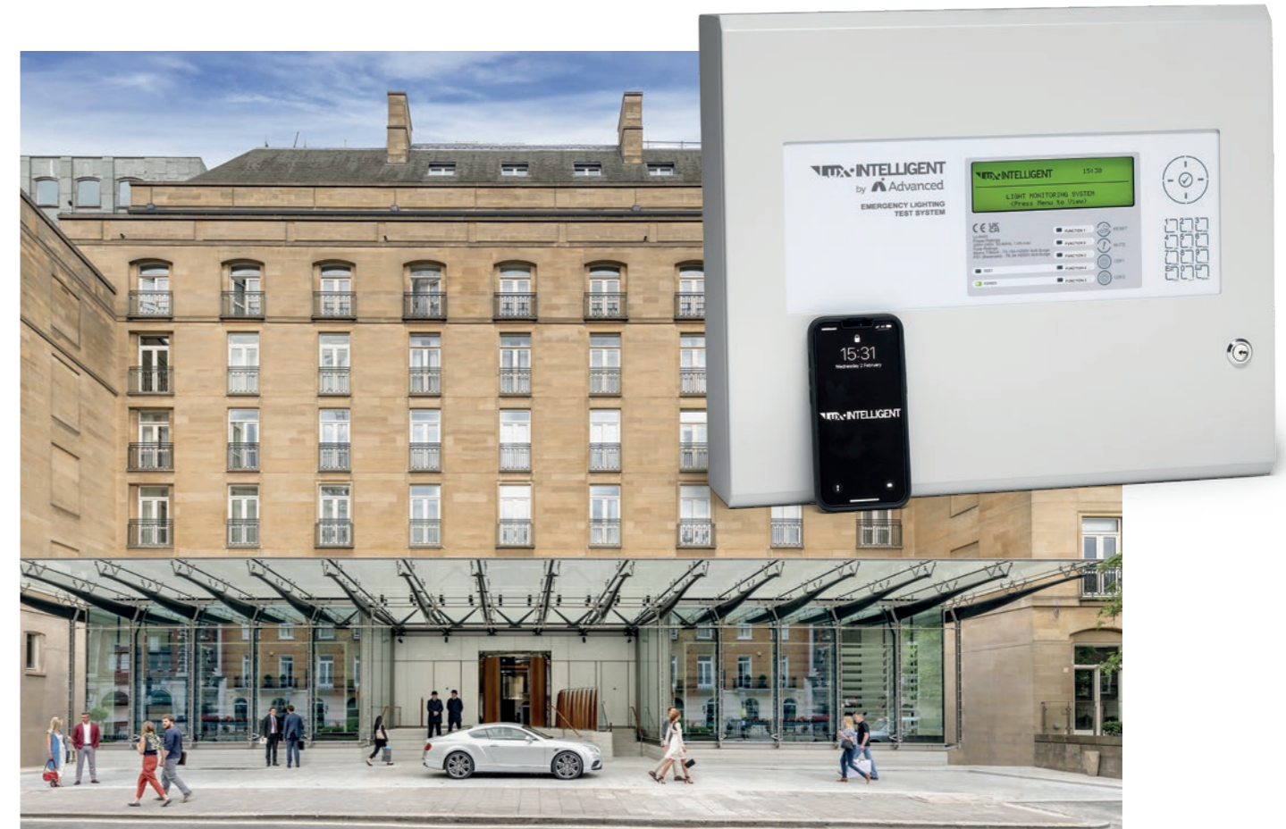
A LuxIntelligent emergency lighting test system was chosen to protect the Berkeley Hotel in Knightsbridge, London because of its outstanding capabilities, features and reliability.
